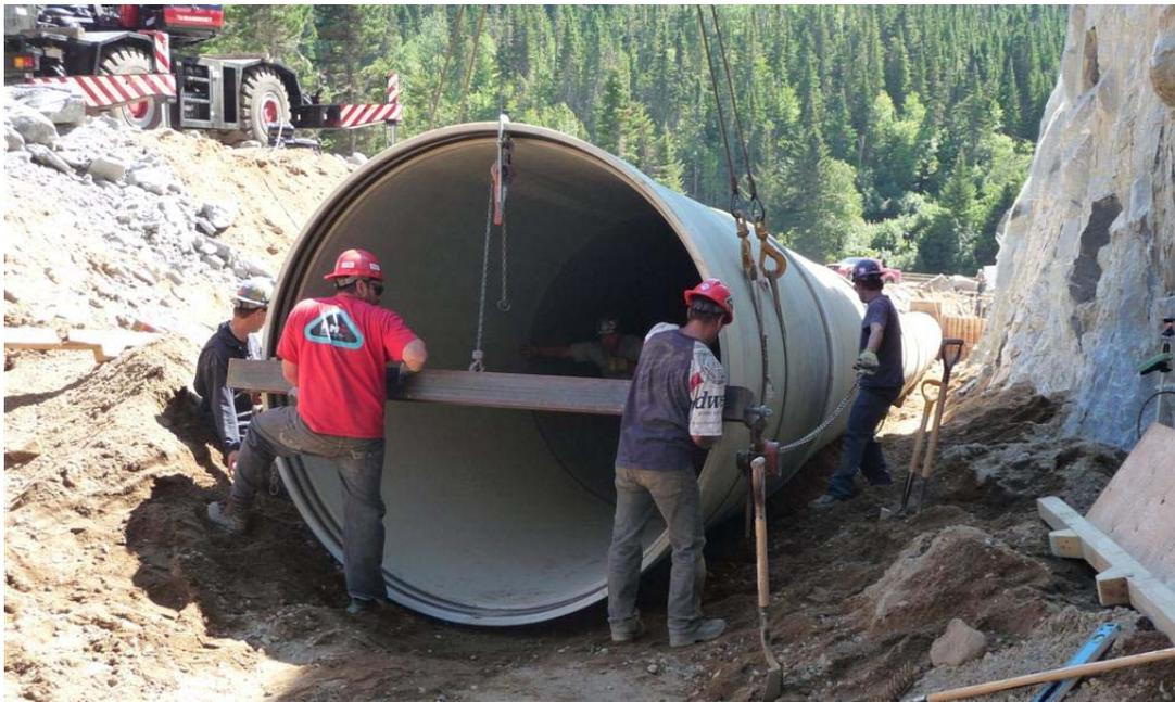
**Figure 6** – Pipe section assembly using Come-a-longs and nylon slings.
