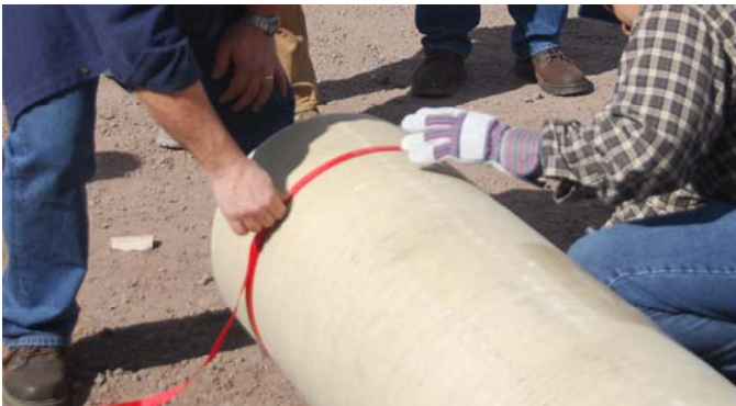
Measure and Mark the Circumference at the Intended Cut Location
