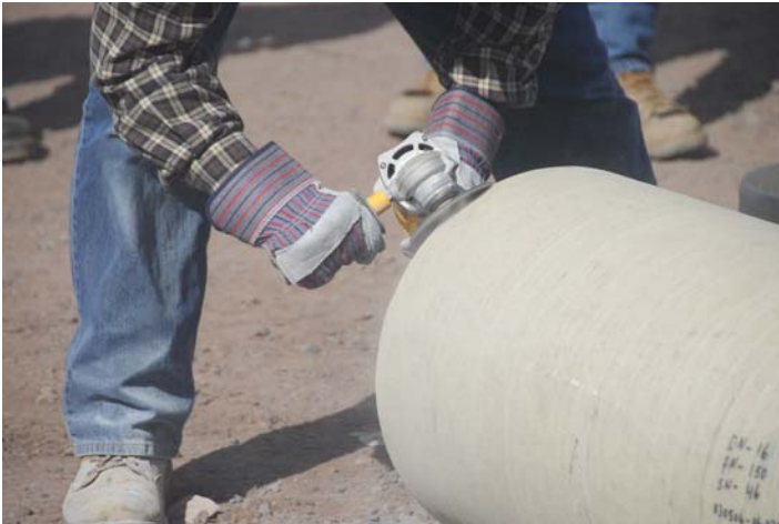
Bevel Cut End for Connection and Clean Cut Surface
