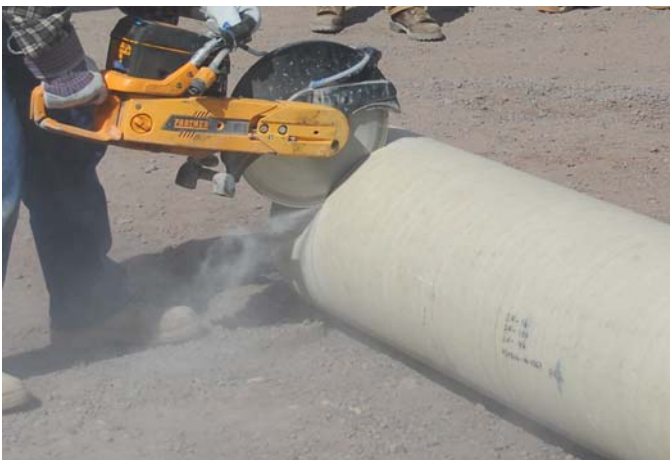
Carefully Cut With A Diamond Coated Blade
